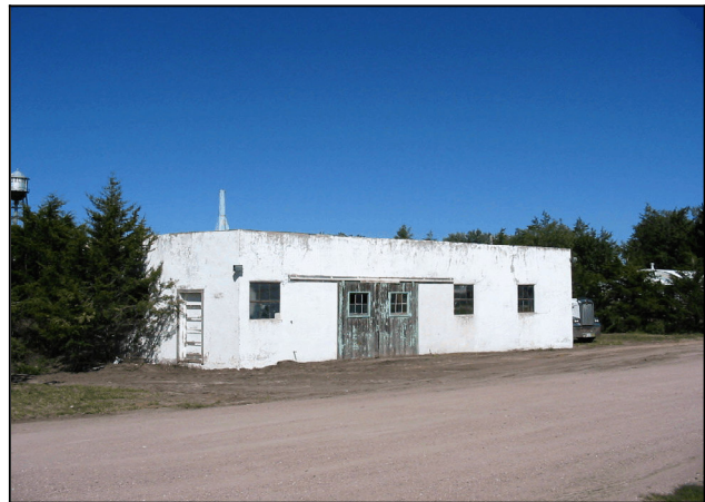
The former Martin Blacksmith Shop building which had been enlarged and remodeled by Cliff Martin in 1940, as it appeared in September 2004 one day before it was demolished to clear the land for a truck parking lot.
